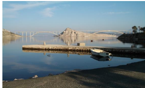
The bridge in Krk
